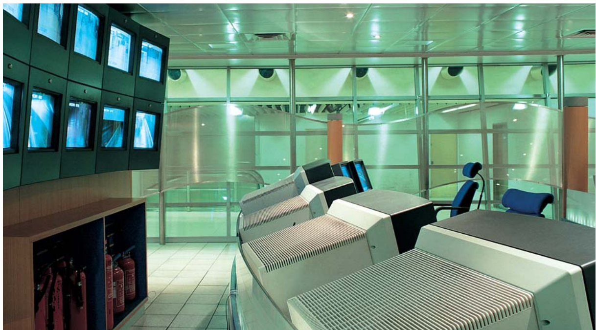
Gare de Lyon, Station RER, Paris/F Lyon station, RER Station, Paris/F
