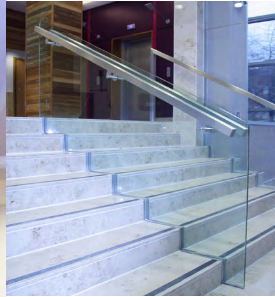
Left: Visually freestanding glass balustrade and applied handrail. Below Left: Nylon system with glass infill. Below Right: Stainless steel handrail and balustrading with glass infill.
