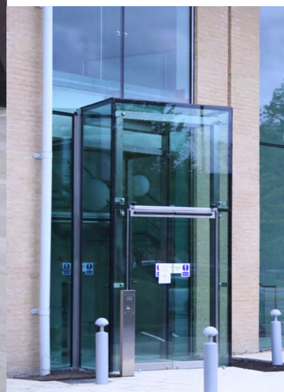
Top Left: Overhead glazing on primary steelwork. Top Right: Underlit laminated glass floor panels with sandblast finish. Above & Left: Bespoke glass entrance and facade on glass fin supports.
