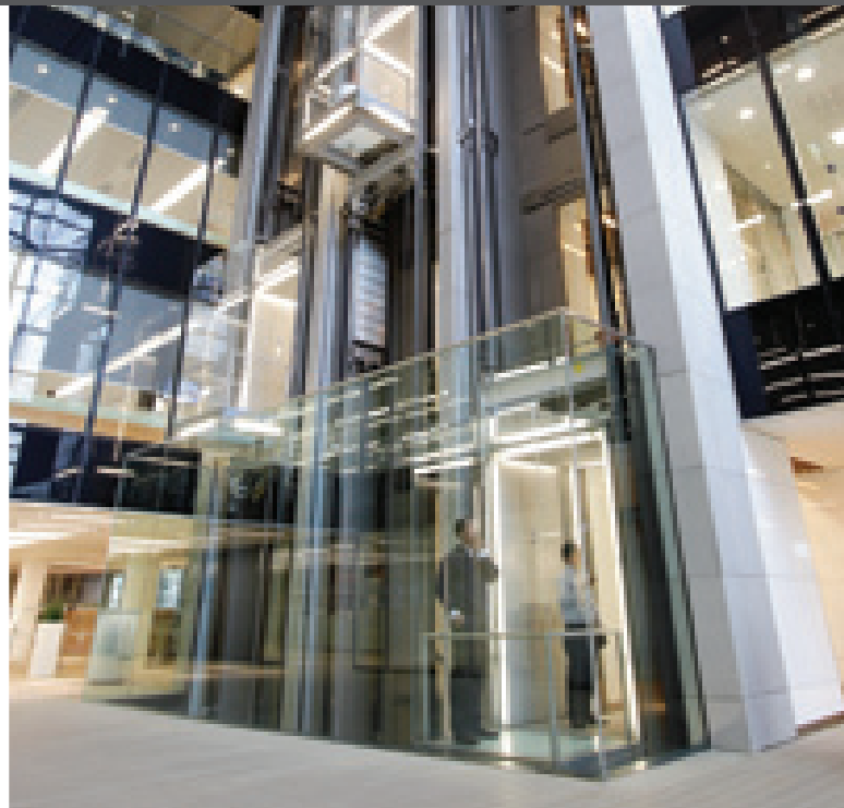
Glass screens around lift shafts, Nomura
