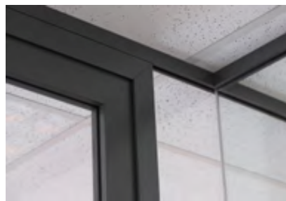
Single Glazed with Applied Kross Glaze Bars
